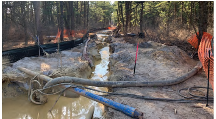
SRL Construction in Manchester April 2019
