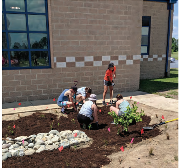
Hammonton High School rain garden installation.
